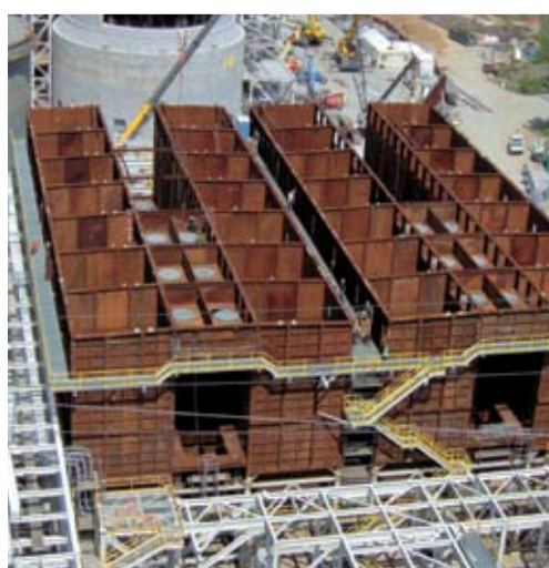
Dominion Power-Chesterfield, Seal welding inside units and floors.
